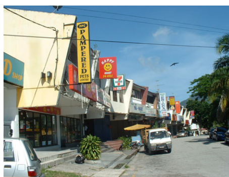
Houses and shops at Tanjung Bunga, MPPP
